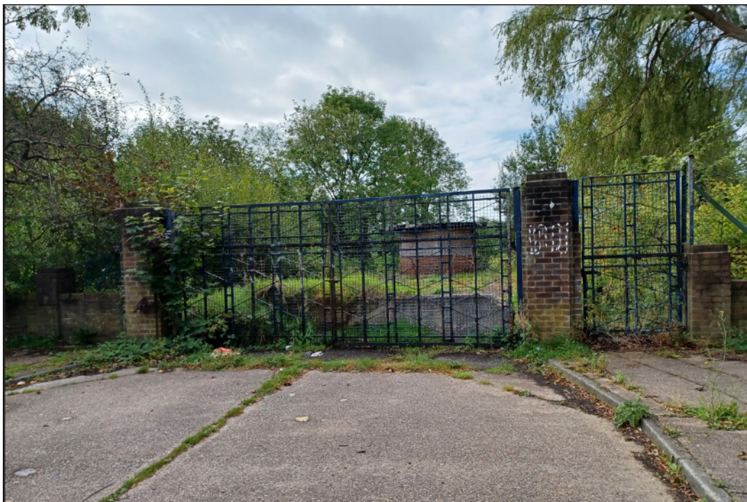
Existing access to the site which would be upgraded
